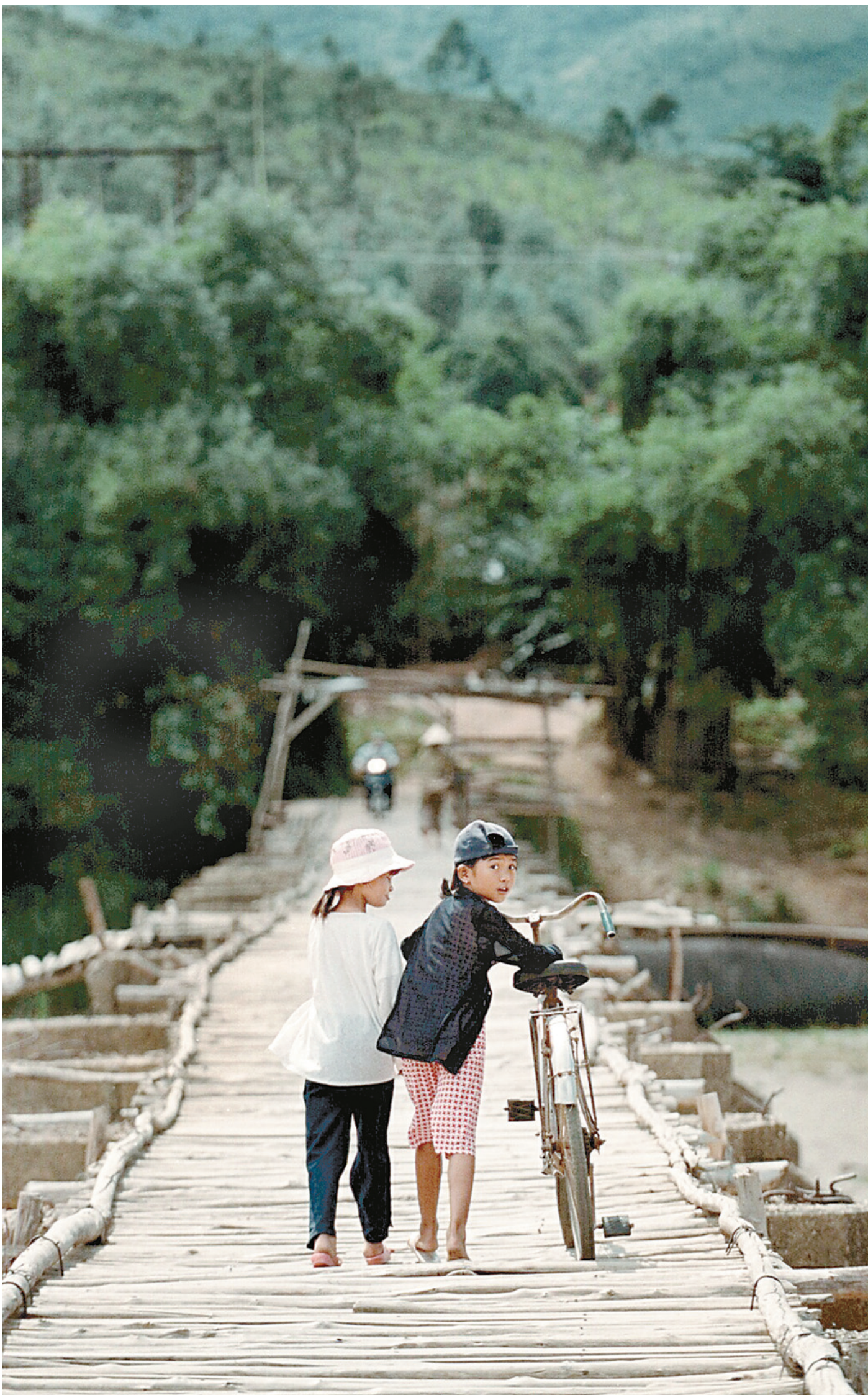
A handmade toll bridge spans the Song Ve River in the Quang Ngai Province of Vietnam. Rural lifestyles are changing, however, and the bridge is slated to be replaced with a concrete span.
